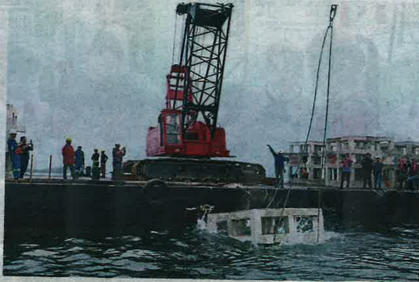
Johor Fisheries Department deploying artificial reefs near Pulau Mertang, Mersing, as part of efforts to protect the marine habitat
