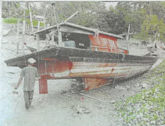
A fisherman repairing his boat at Pengkalan Tangkiah. Regular maintenance is crucial to ensure the boats do not sporting a leak. — Photos: GRACE CHEN/The Star
